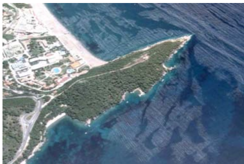
Cape Zavala before initiation of construction
